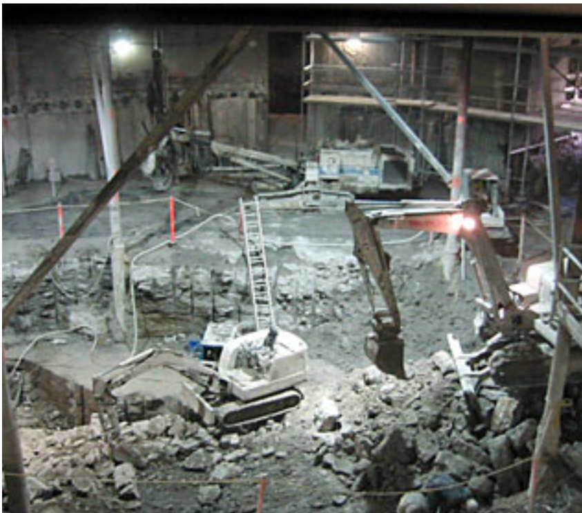
Excavation work continues in basement levels.
