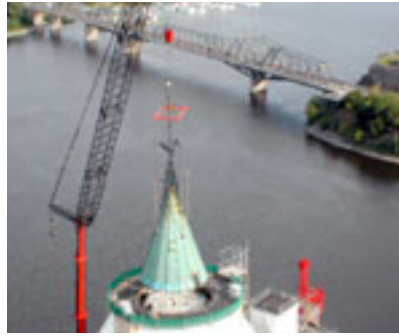
Upper roof structure and weathervane lifted from the Library of Parliament building.
