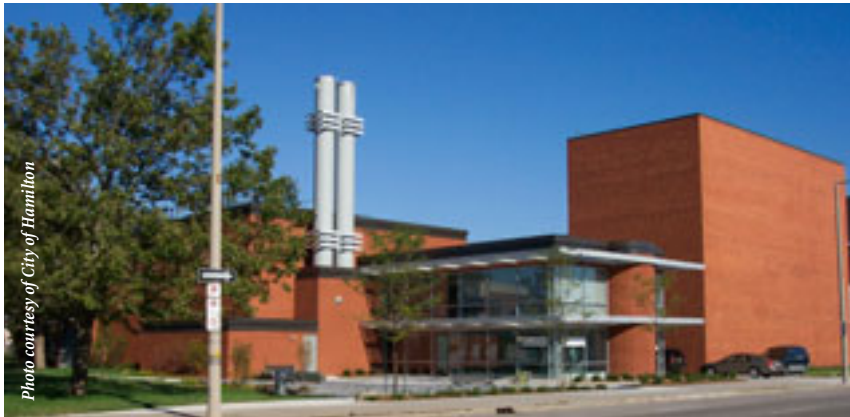
Hamilton Community Energy Plant.
